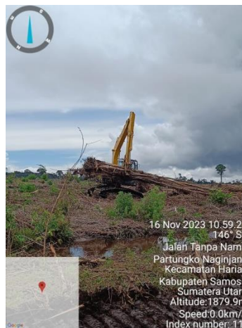
Gambar 1. Proses Extraction Excavator Grapple
