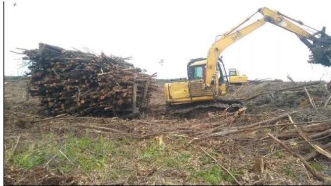
Gambar 2. Proses Extraction Excavator Ponton Darat
