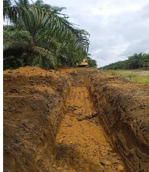
Gambar 4.6 Parit pengaman 2 x 2 x 1 m
