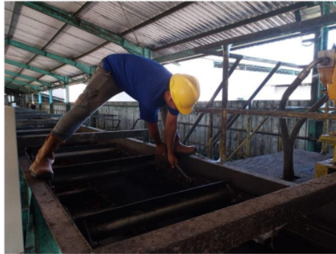
Gambar 1. Mekanik Preventive Baut Chain Screper Conveyor No 2
